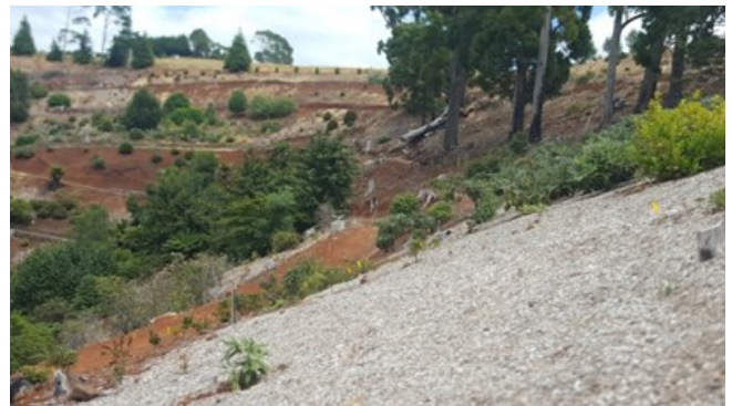
Photo 2- result of spraying and mulching.
