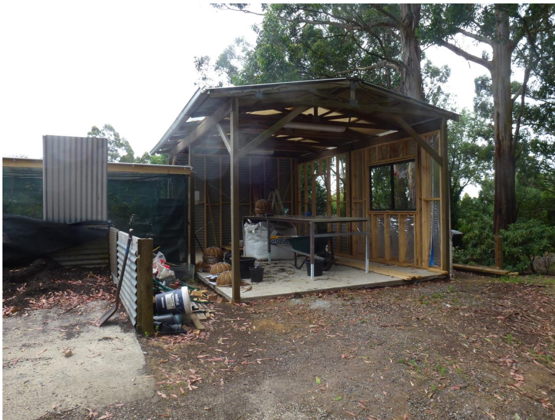
New Potting Shed, NRG, construction by John O'Hara and Michael Hare
